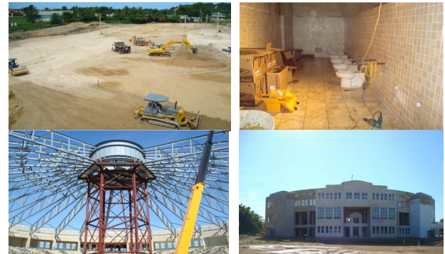
Coliseum of Aguada under construction
